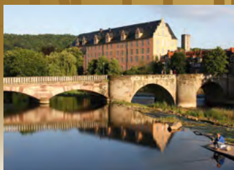
Hann.Münden, Werrabrücke bridge (Photo: Hann. Münden Marketing GmbH)
